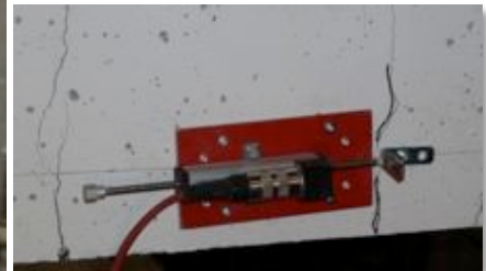
LVDT measuring Crack Width
