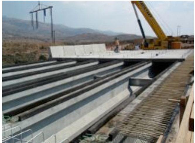
Utah DOT – Emma Park Bridge Precast Deck Panels
