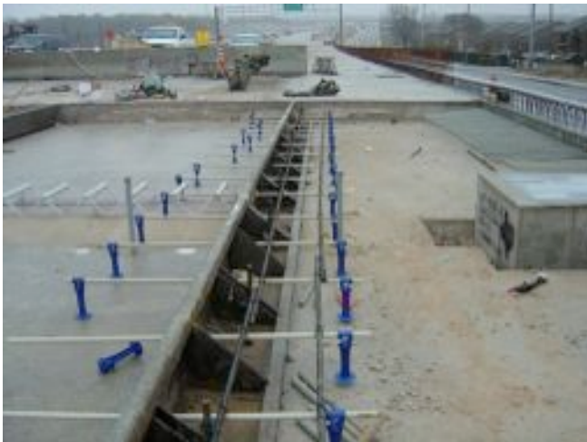
Texas DOT – High Speed Tolling – Tie Bars
