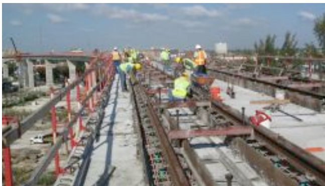
Miami MetroRail – Concrete Plinths for electrical isolation
