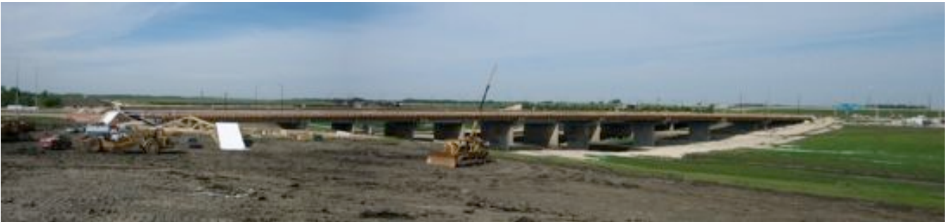
Floodway Bridge – Winnipeg, Manitoba
