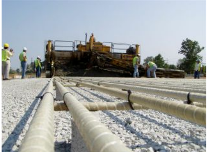
West Virginia – CRCP Paving
