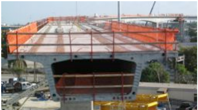
Miami MetroRail – Deck Bars for electrical isolation in Segmental Precast
